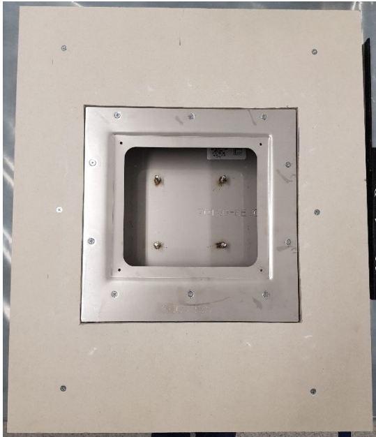
Image 2 - Mounting of Joramark Box300 in a plasterboard
