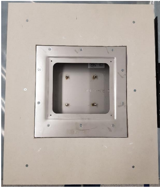
Image 2 – Mounting of Joramark Box300 in a plasterboard
