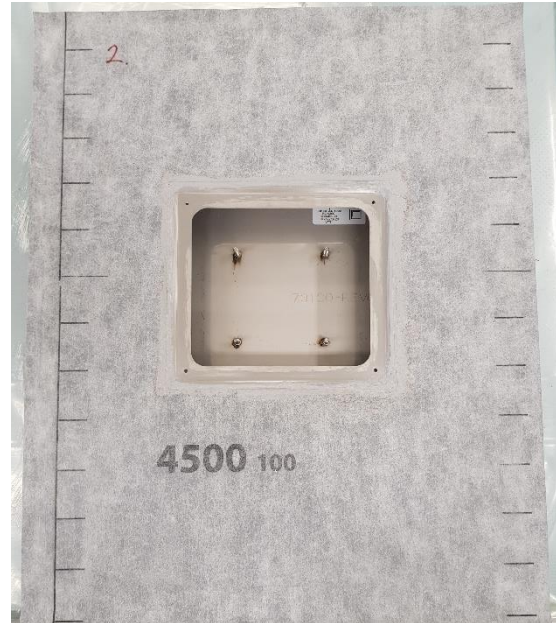
Image 4 – Mira Vapourmat 4500 applied and the edges sealed with Mira 3690 One-seal
