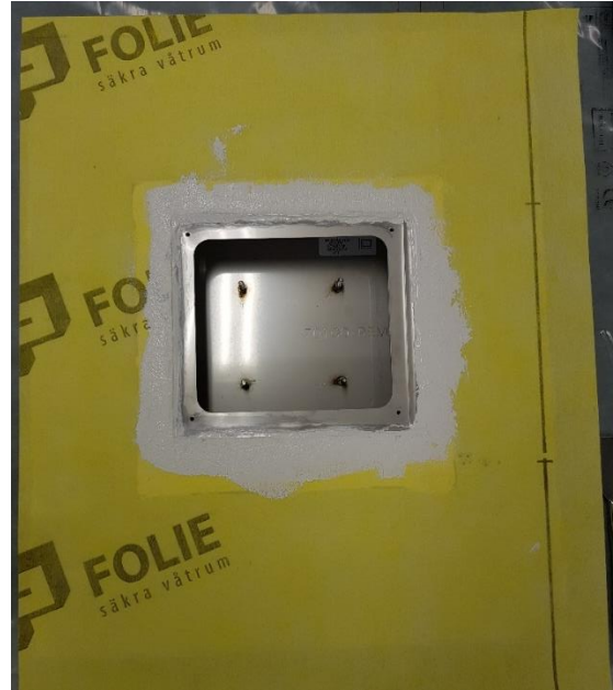
Image 4 - LIP Foile G3 applied and the edges sealed with LIP skarvlim MSP
